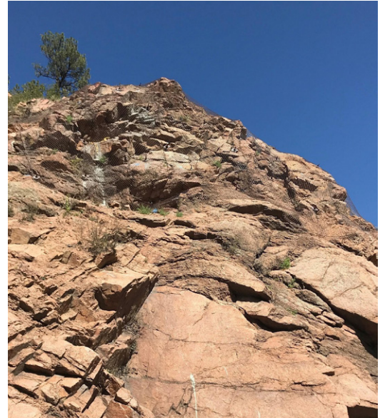
Exhibit DS22.1: Anchored mesh installed on US 24 Ute Pass.
