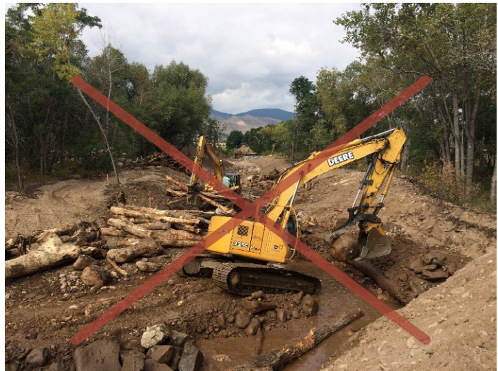
Exhibit P7.6: Example of tree and vegetation removal.
